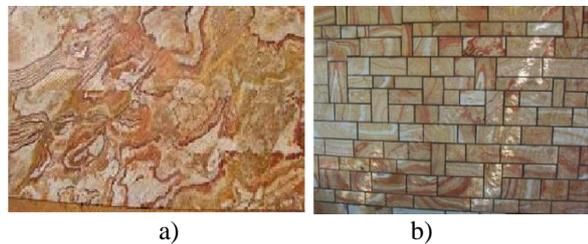
Fig 3. Application areas of Çan stone a) Patterned structure, b) Exterior cladding [11]
